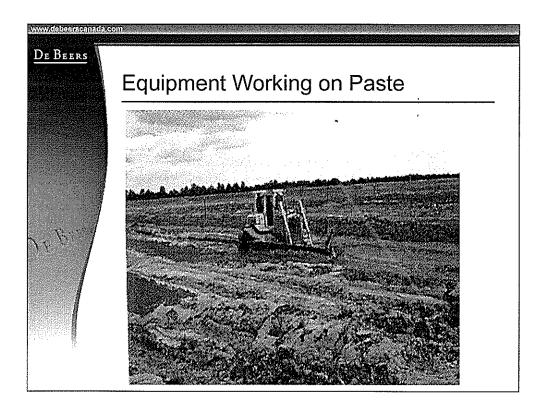
After paste has been on the surface for a short time, anywhere from a few days to a few weeks, if it does not freeze, it will consolidate. In either case, whether frozen or consolidated, equipment will be able to work on the surface. This will allow the cap to be placed a short time after an area is completed.
