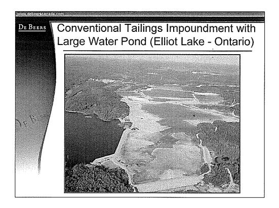
This is a photograph of a tailings facility that uses slurry deposition. This type of system has been used throughout the north, for example at Colomac, where you can see the large permanent ponds that are part of the operation.
