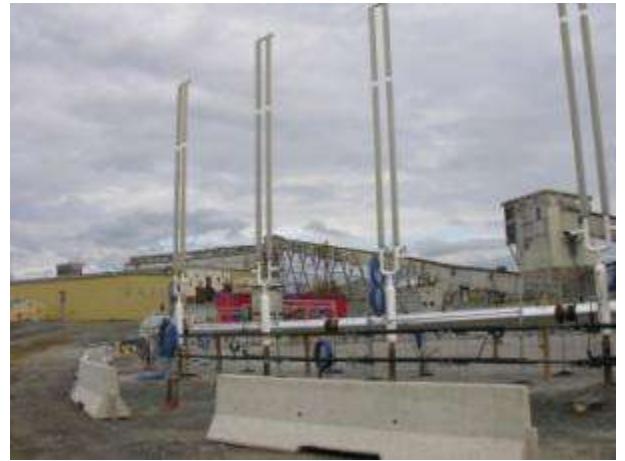
Giant Mine thermosyphons
