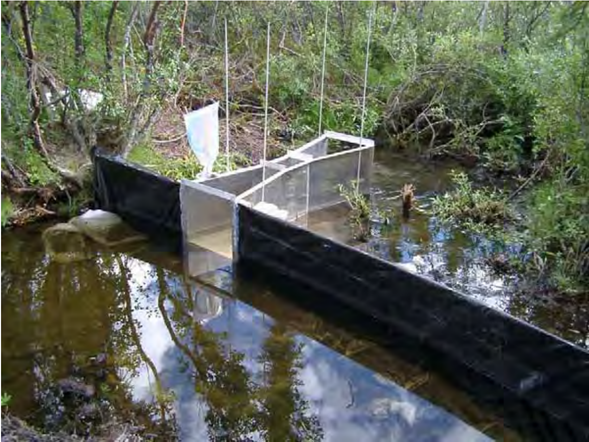
Site#4: Hydrometric Gauging Station With installed Parshall flume
