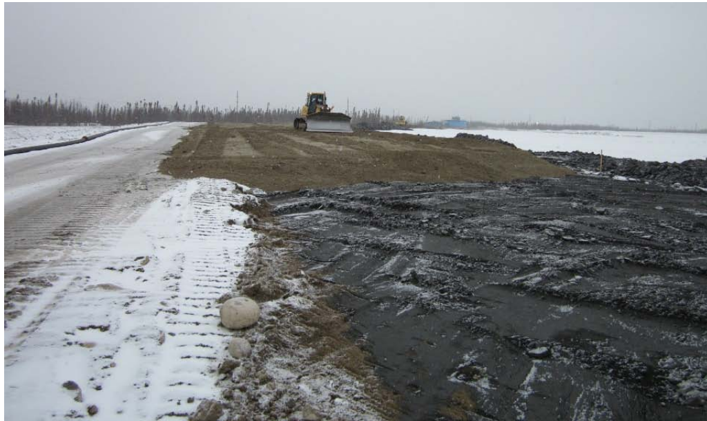
Photo 31: Typical Raise 1 Discharge Dyke Construction without Geogrid over Thickened Tailings
