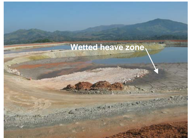
Photo 11: Completed Type 1 Co-disposal Pad
