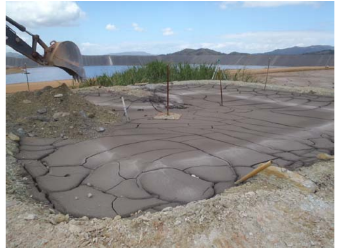
Photo 24: Placing PAG mine rock lift over cell with 2 m depth of tailings
