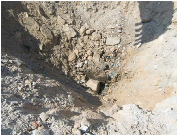
Photo 16: No standing water after excavation, indication tailings displacement
