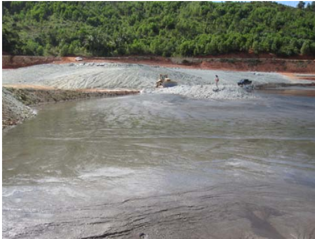
Photo 14: Advancing containment berms out into freshly deposited thickened tailings
