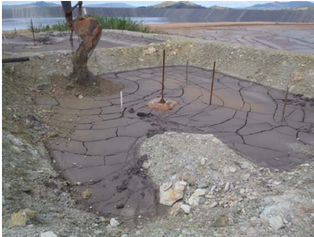
Photo 23: Placing PAG mine rock lift over cell with 1m depth of tailings
