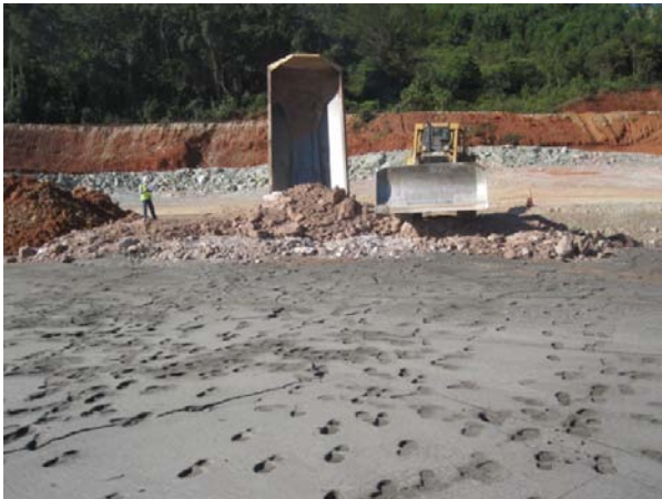
Photo 10: Spreading PAG mine rock over desiccated thickened tailings beach
