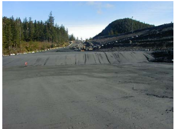
Photo 7: Greens Creeks Compacted Surface of Co-mingled Surface
