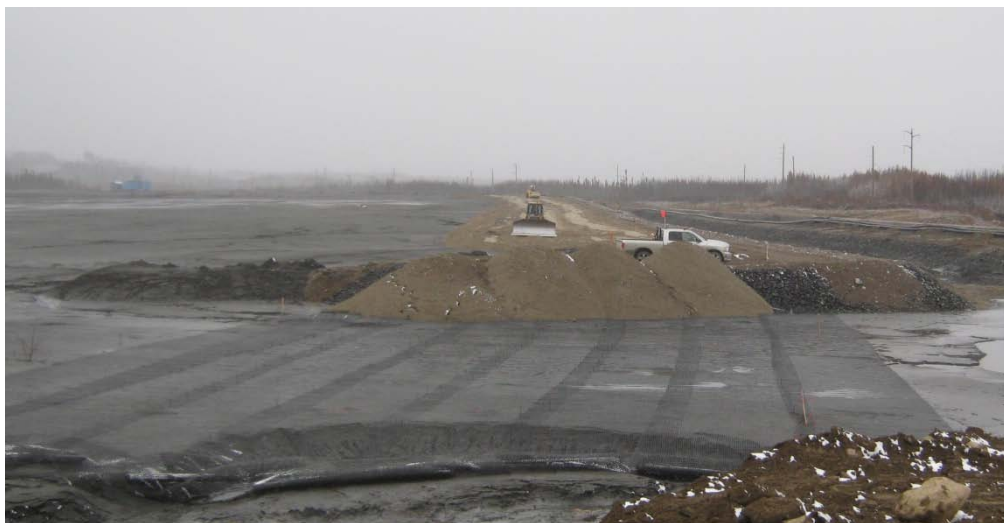
Photo 30: Typical Start-up Discharge Dyke Construction with Geogrid over Soft Tailings Slurry
