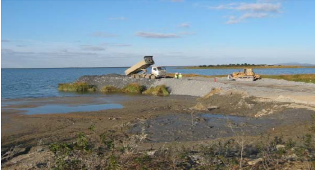
Photo 1: Truck off-loading mine rock and dozer spreading at Neves Corvo
