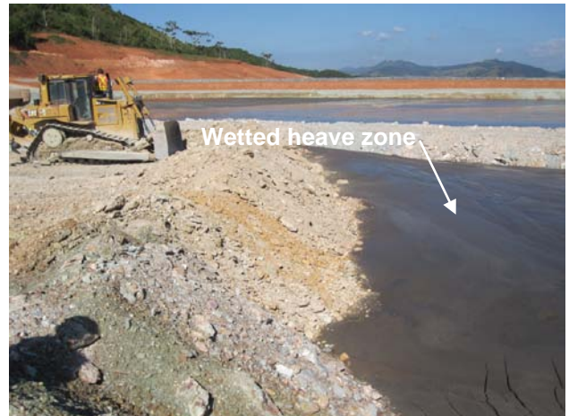
Photo 15: Spreading PAG mine rock over freshly deposited thickened tailings
