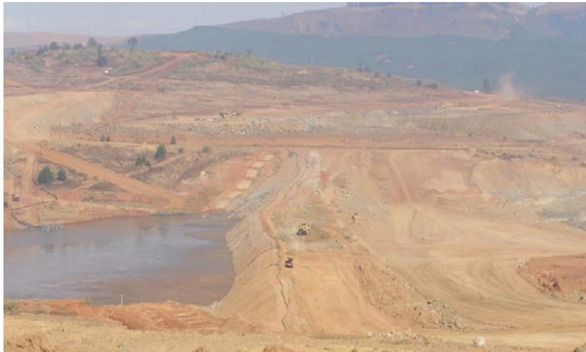
Photo 26: South African Tailings Slurry and Overburden Waste Co-disposal Facility Construction
