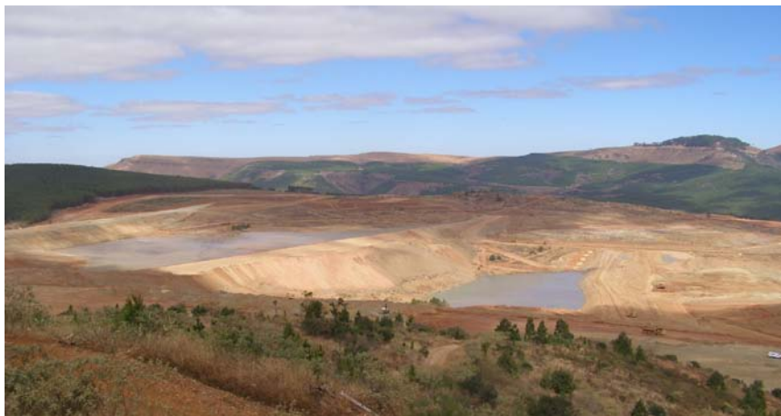
Photo 25: South African Tailings Slurry and Overburden Waste Co-disposal Facility
