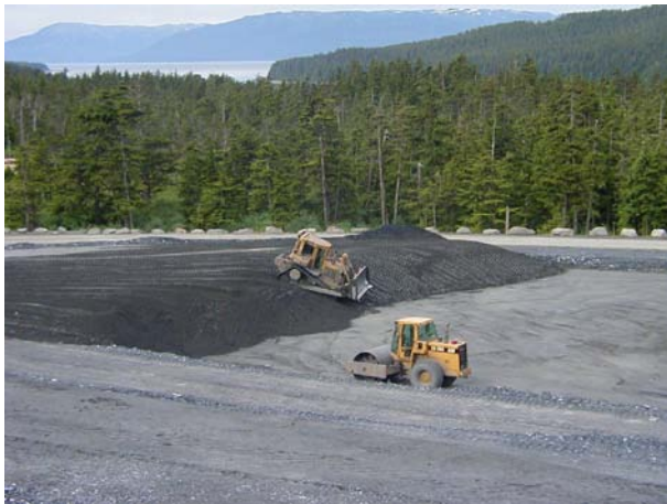
Photo 6: Greens Creeks Co-mingling of Filtered Tailings and Miner Rock
