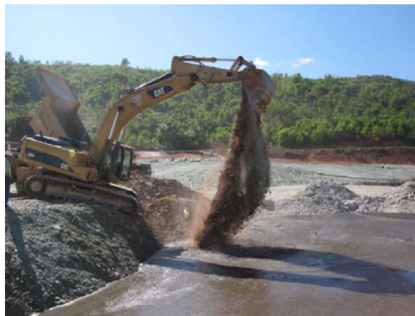
Photo 18: Dropping PAG mine rock into freshly deposited thickened tailings using an excavator
