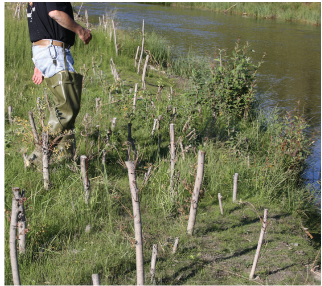
figure 30. Willow plugs can be planted to control erosion in sensitive areas such as riparian zones.
