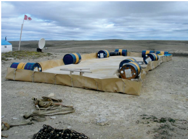
figure 18. Secondary containment structures can also be used for fuel drum storage.
