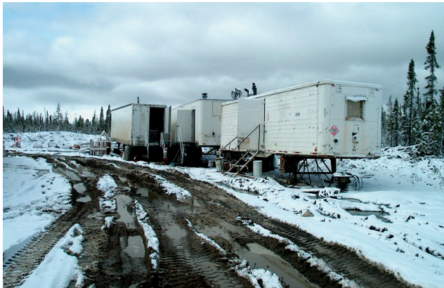
figure 13. Deep rutting and soil erosion can occur if operations continue too late in the spring.
