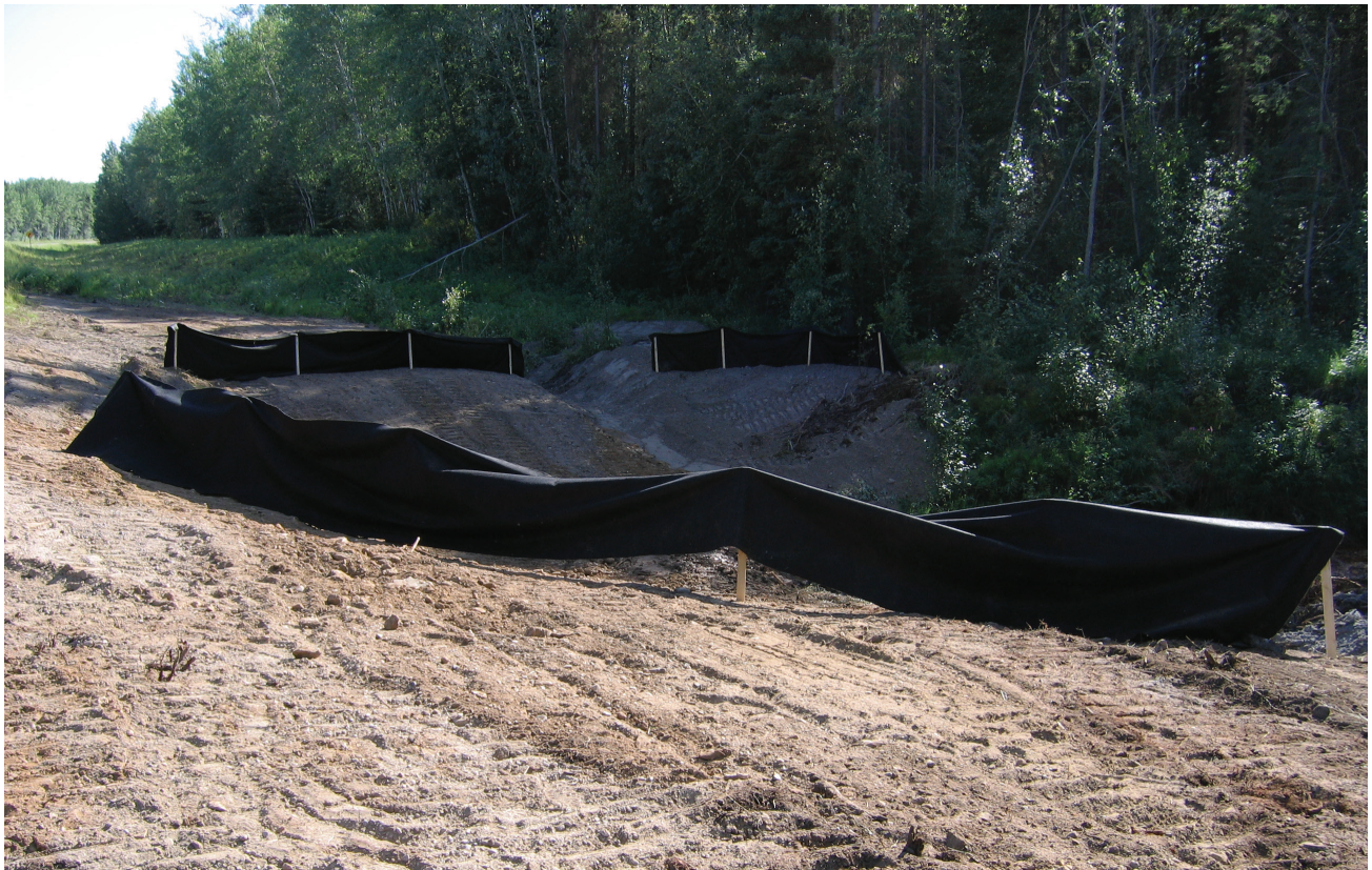
figure 17. Sediment curtains used for drainage control at the edge of a clearing.
