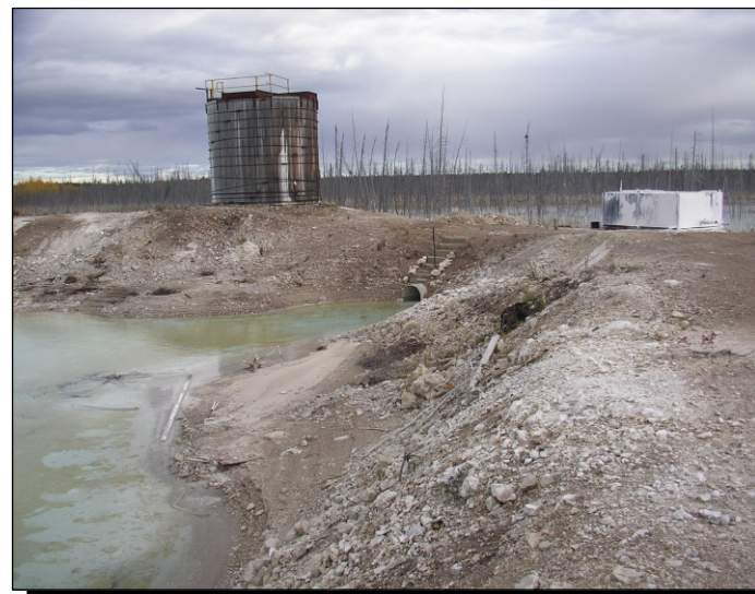
Photo 8 Water Station 7 Pine Point Tailings Pond.
