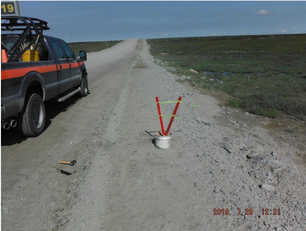
FIGURE 4. THE STAKED BUFFER AREA LOCATIONS FOR THE ENVIROKLEEN APPLICATION ON SABLE ROAD, 2019
