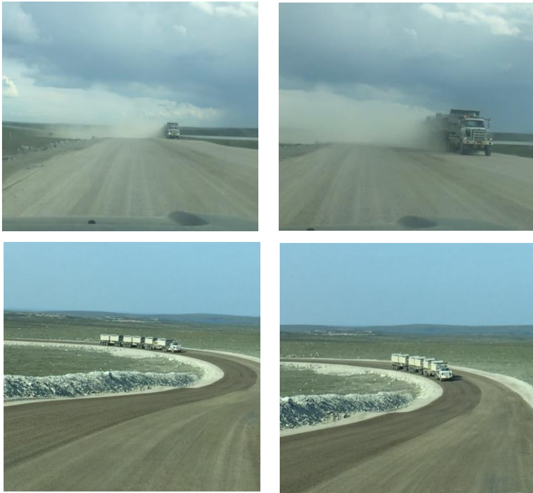
FIGURE 19. VIDEO OBSERVATIONS OF DUAL POWERED ROAD TRAIN VEHICLE BEFORE (TOP PANEL) AND AFTER (BOTTOM PANEL) ENVIROKLEEN MAINTENANCE APPLICATION ON SABLE ROAD, 2019
