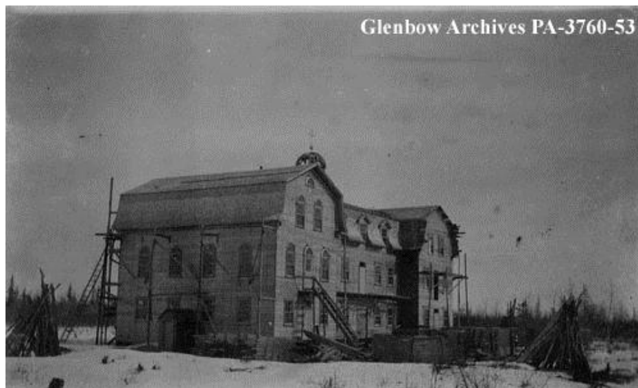
Plate 39: Roman Catholic mission under construction, Fort Resolution 472
