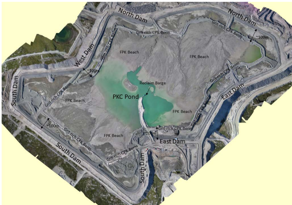
Figure 4: Processed Kimberlite Containment Facility
