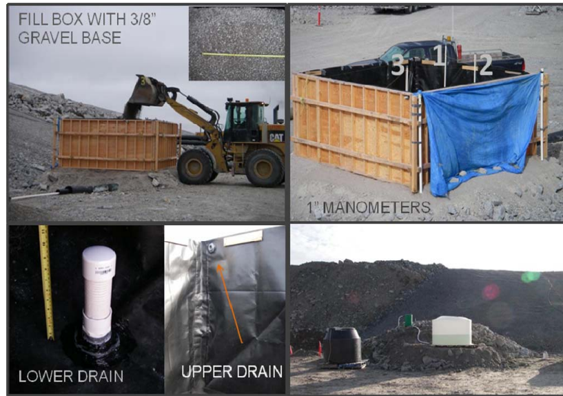
Figure 2-17. Construction of 32 m 3 field permeameter experiment.
