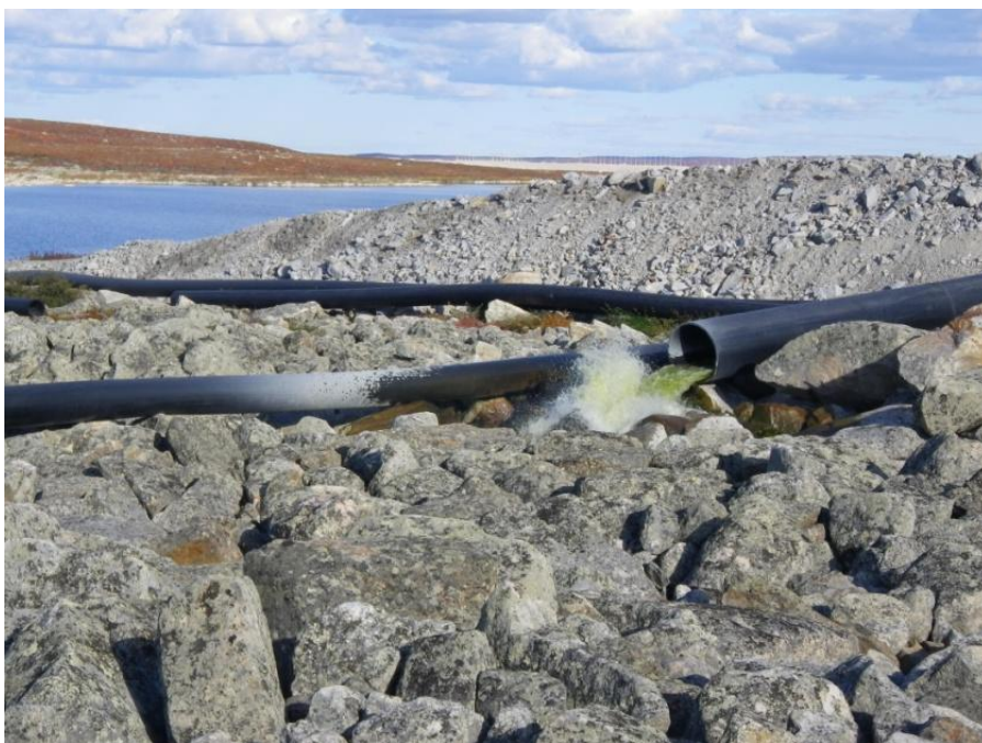
Figure 4: Second discharge pipe to North Inlet from direction of NIWTP. Discharge water contains green suspended material, presumed to be algae. UTM coordinates (UTM Zone 12): 533672 easting, 7153536 northing.
