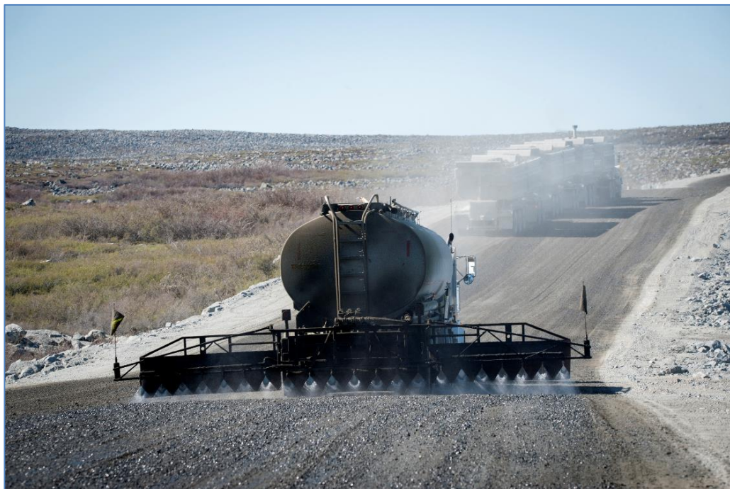
Application of dust suppressant, Misery Road, undated.
