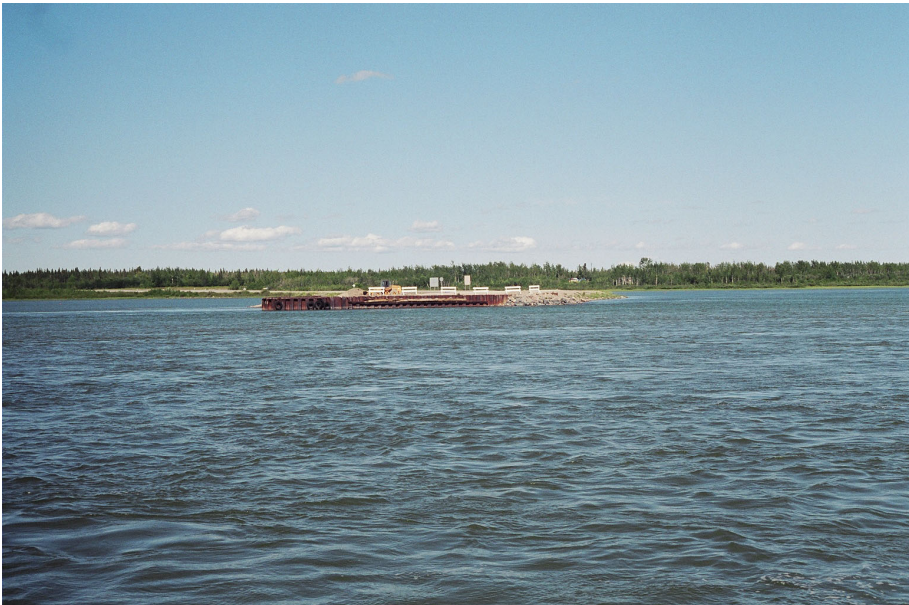
Plate 3 30 July 2003. View of main channel and steel plate armouring on nose of north causeway.
