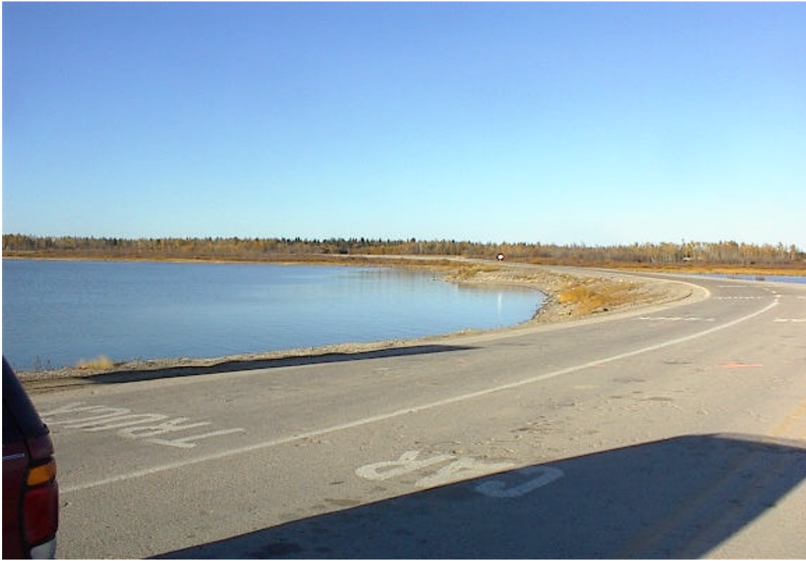
Photo 3: Looking northeast from southern end of northern ferry landing.
