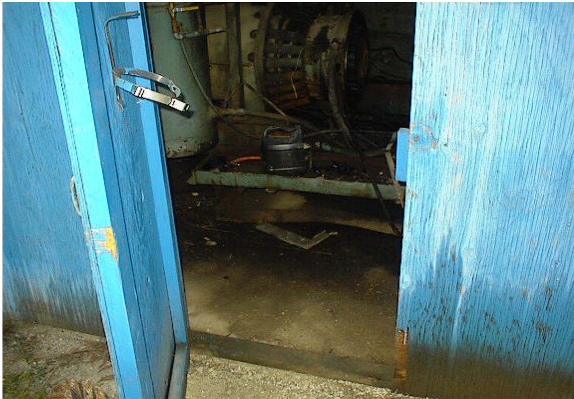
Photo 20: Concrete floor inside gear house.
