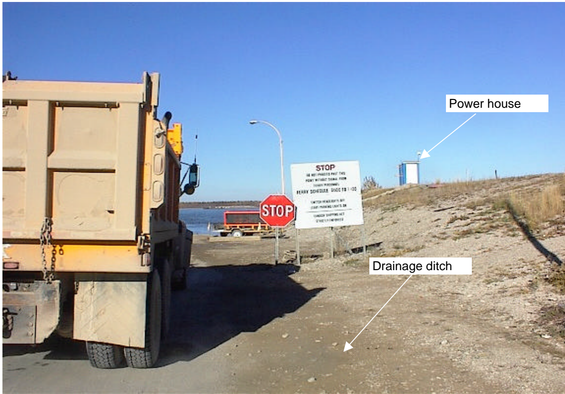
Photo 9: East side of southern landing looking north, power house for lights located on top of berm.
