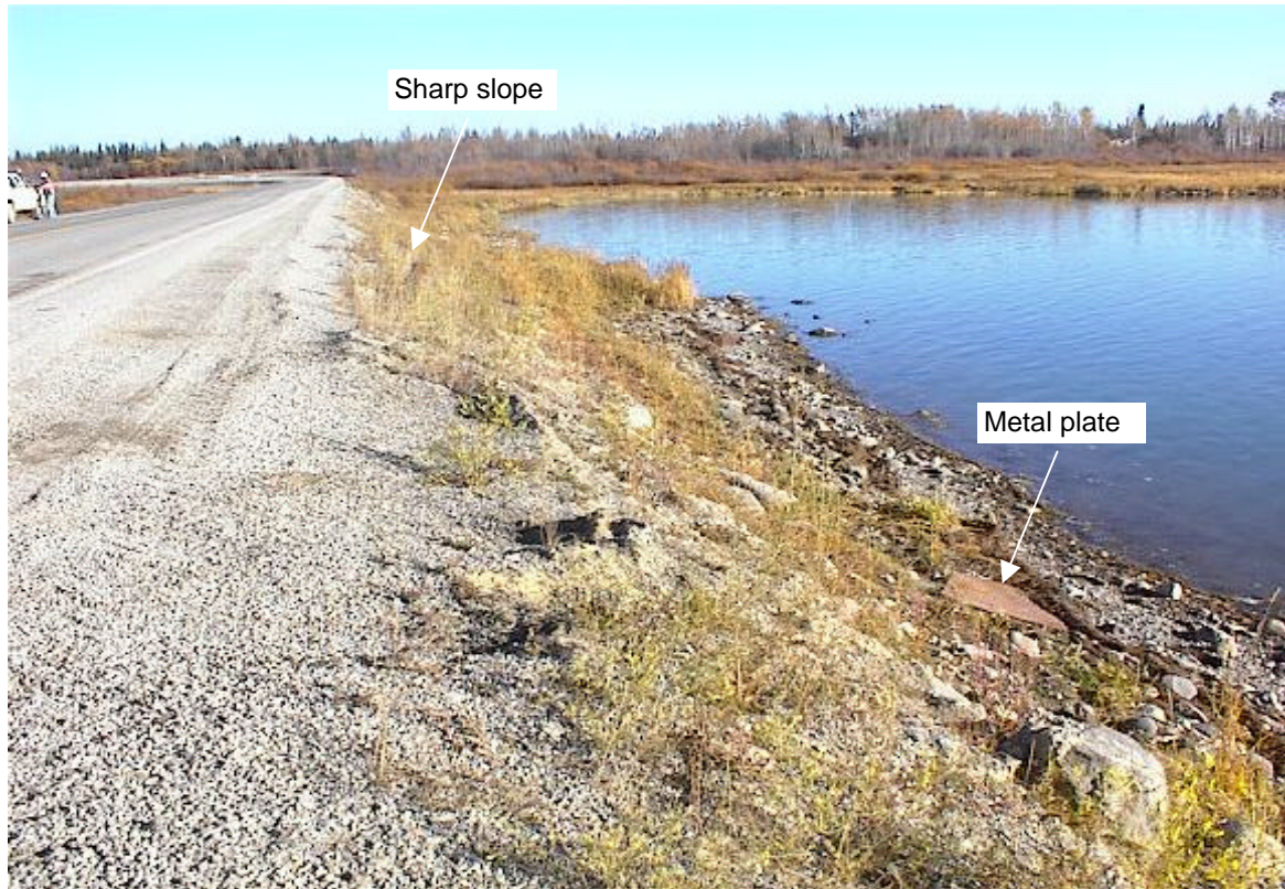
Photo 2: Looking north along eastern edge of northern ferry landing.
