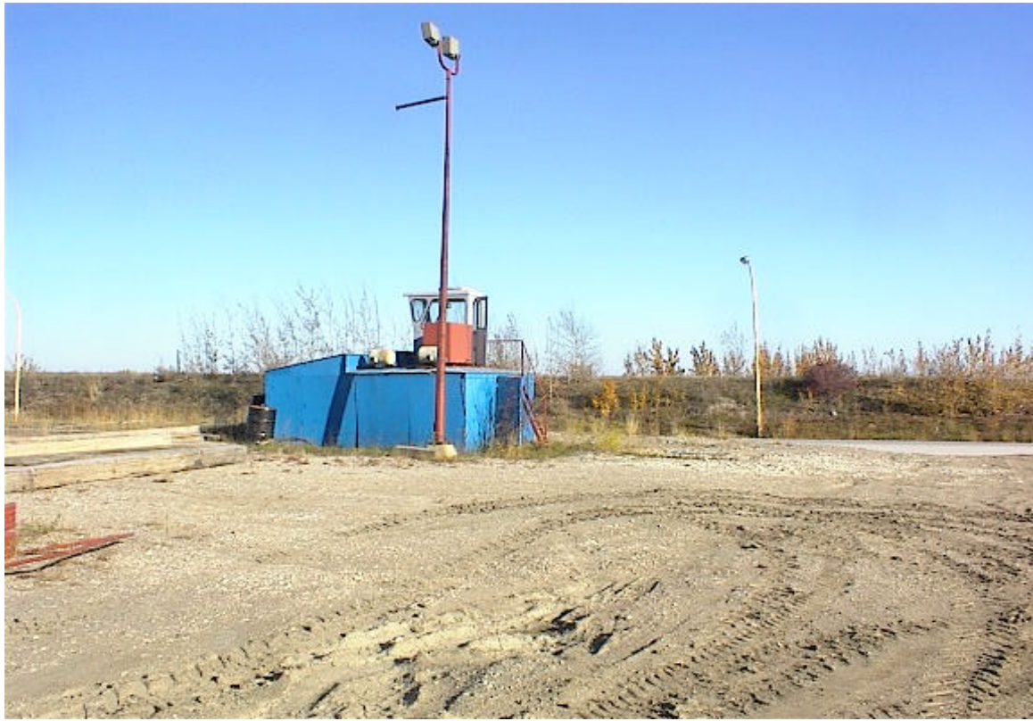
Photo 13: Southern landing looking east at eastern winch house.
