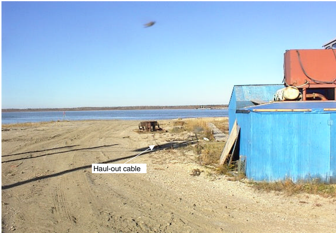
Photo 12: Southern landing looking north, western winch house on left.
