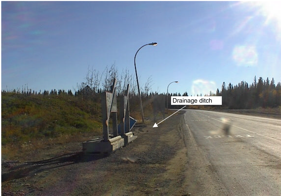
Photo 10: Drainage ditch on east side of southern landing looking south.
