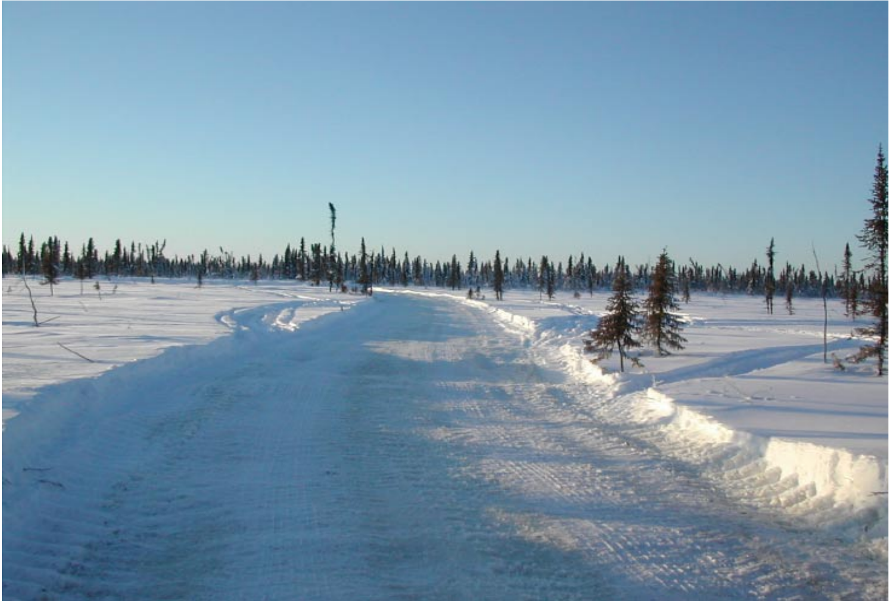
Access: Six-metre access trail construction – GSA Winter 2004
