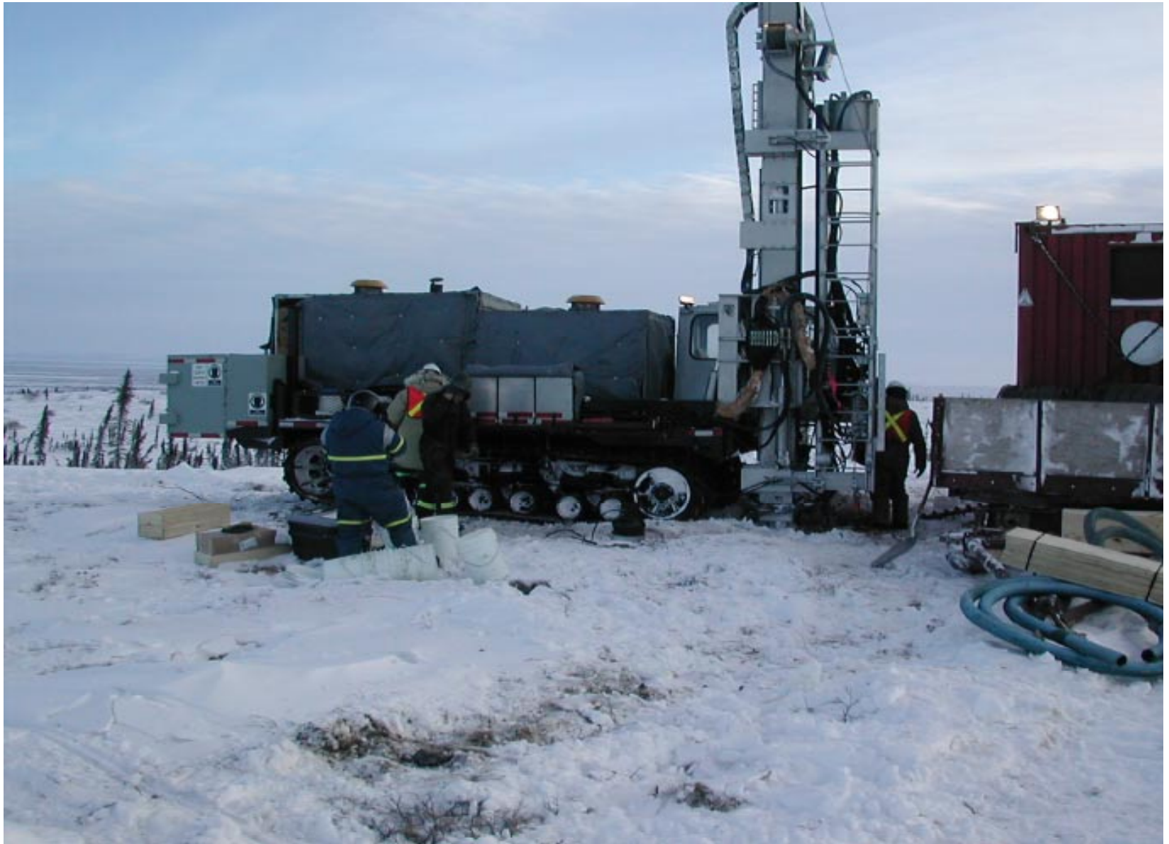
Operations: Drill rig setup at borrow site – GSA Winter 2004
