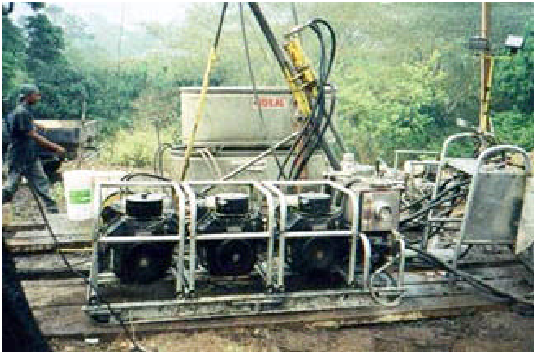
Plate 3: Typical modular helicopter portable drill rig.
