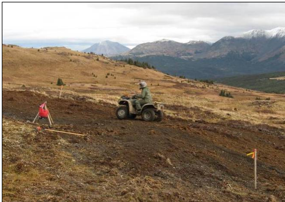
Photo 8 – Drill pad scarification with quad-towed harrow
