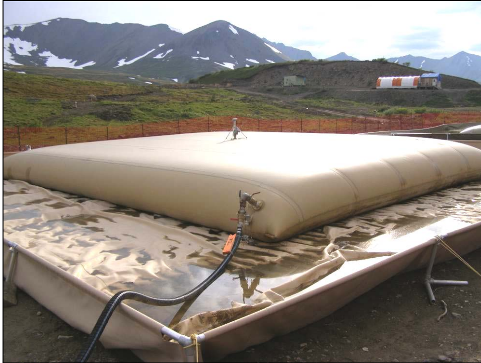
Photo 3 – Arctic Guard tank with secondary containment
