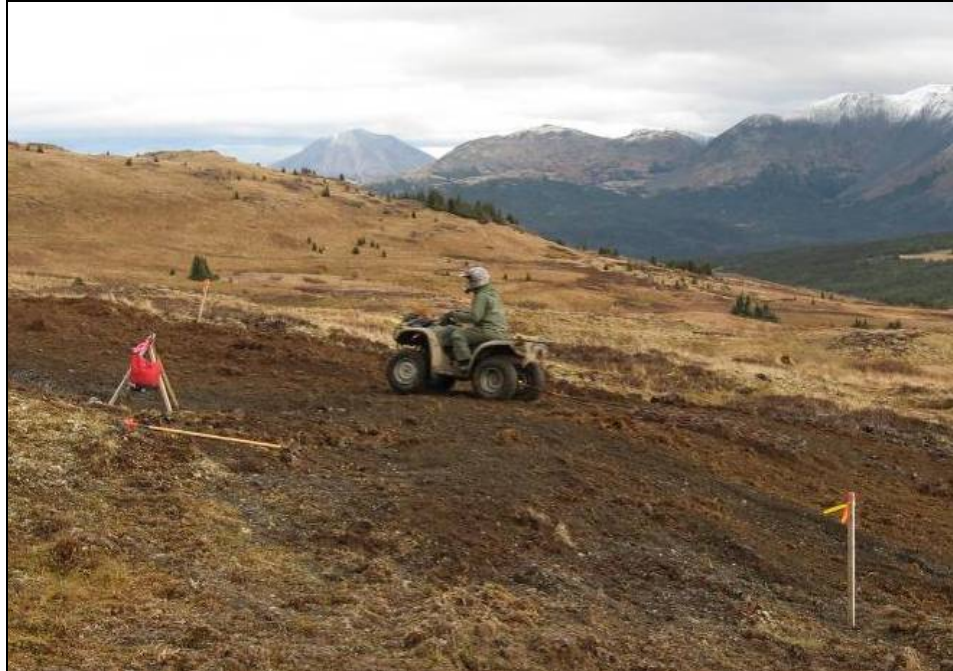
Photo 8 – Drill pad scarification with quad-towed harrow
