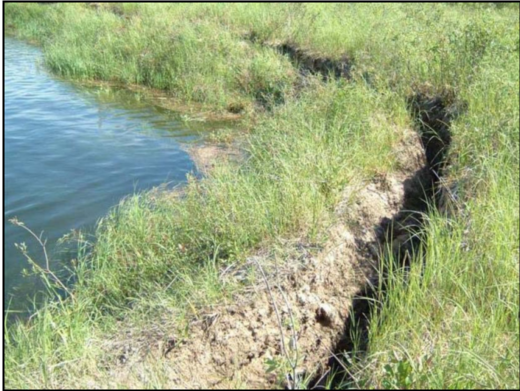
Plate 14.4.1 — Tension Cracks at Site 1
