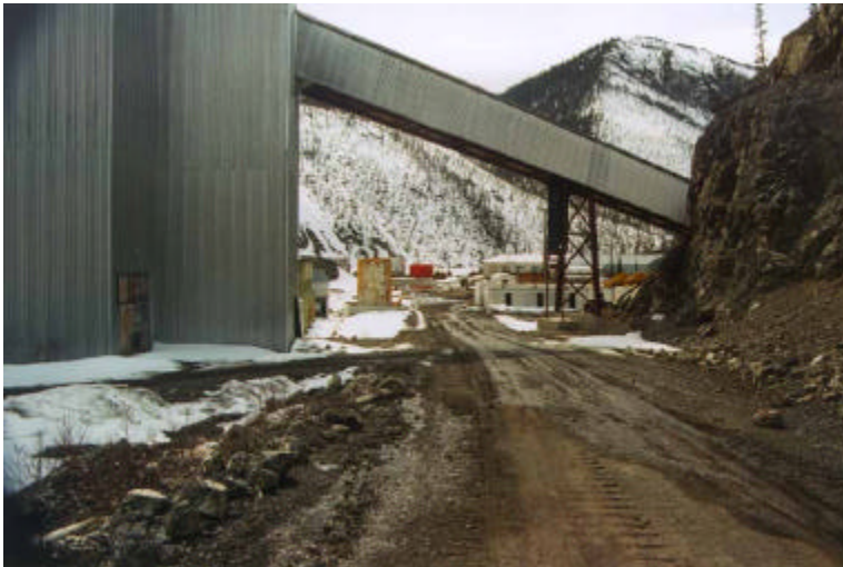
Coarse Ore Conveyor Gallery – View Towards Shops and Camp
