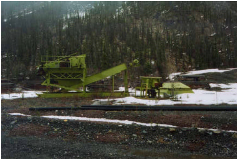
Portable Sand Wash Plant – Located Beside Airport Runway
