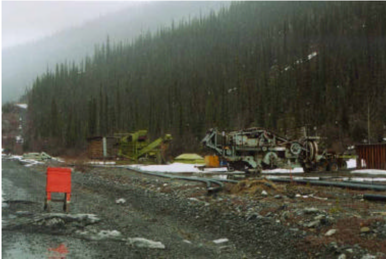
Portable Cedar Rapids Crusher - Located Beside Airport Runway
