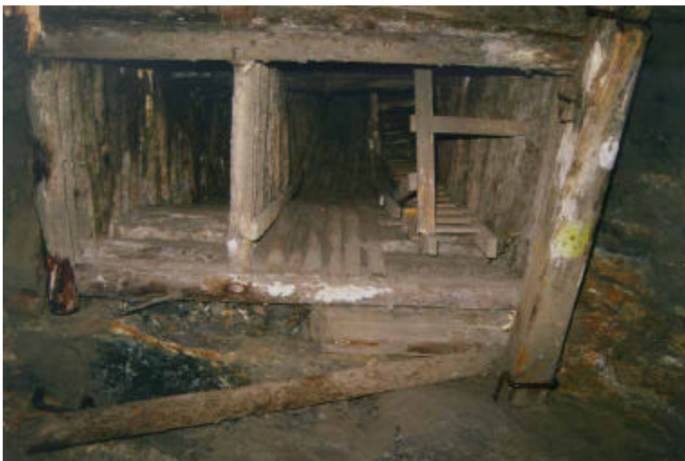
Timber Service raise 930m-870m
