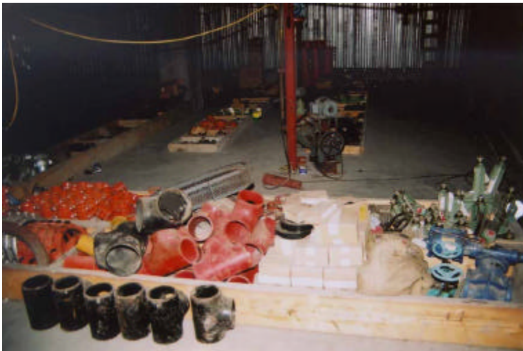
Mill Spares in Basement
