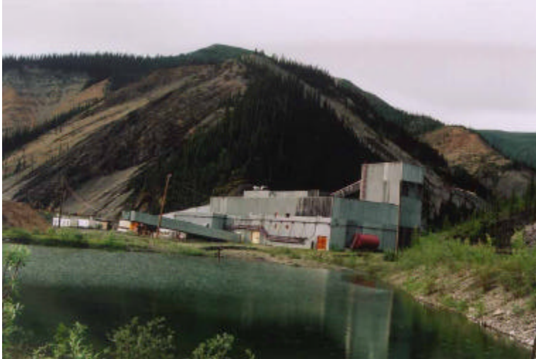
Mill Building from South East
