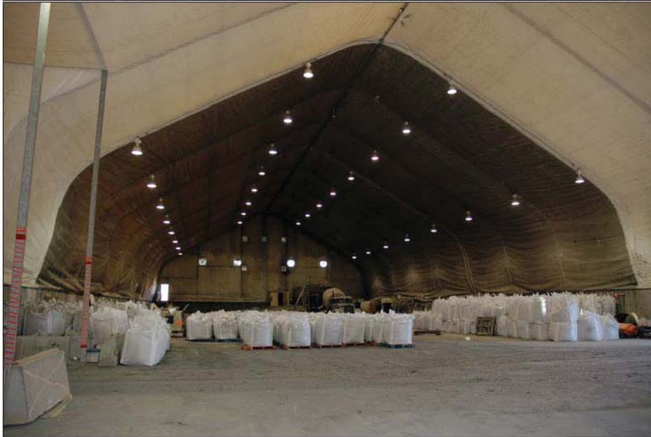
Plate 2: Proposed Structure for Tetcela Transfer Facility TOP: Exterior View of Structure, in place at Ekati Mine BOTTOM: Interior View of Structure Showing Concentrate Tote bags (photo courtesy of Sherwood Copper)
