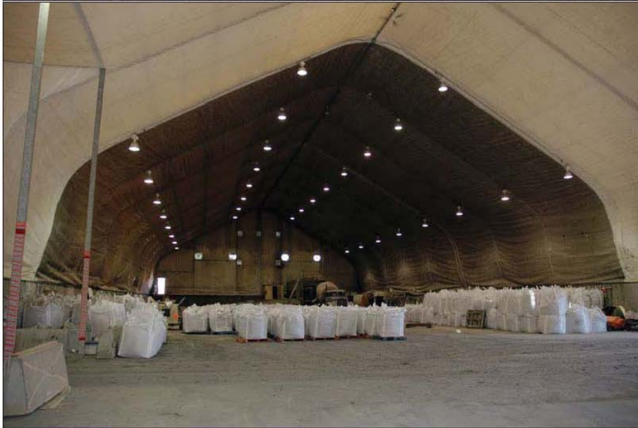
Plate 2: Proposed Structure for Tetecla Transfer Facility TOP: Exterior View of Structure, in place at Ekati Mine BOTTOM: Interior View of Structure Showing Concentrate Tote bags (photo courtesy of Sherwood Copper)
