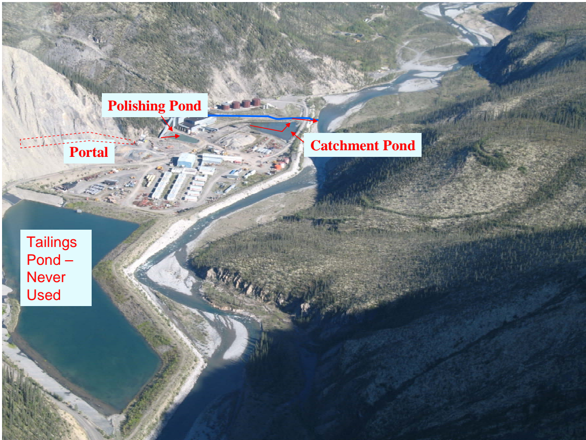
Figure 2. Aerial overview of Prairie Creek exploration property showing portal discharge flowing into the polishing pond then to the catchment pond and into Harrison Creek. Harrison Creek then discharges into Prairie Creek.
