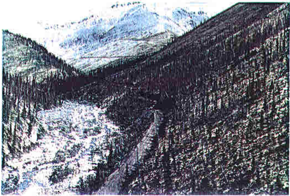
Figure 4: Looking east, Mile 7.2 to Mile 9.0 Km 11.5 - 14.5 under construction (27/07/80).
