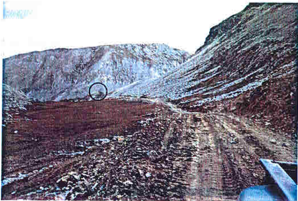
Figure 9: Looking west, Mile 10.3 after road construction (26/08/80). Note point of reference.
