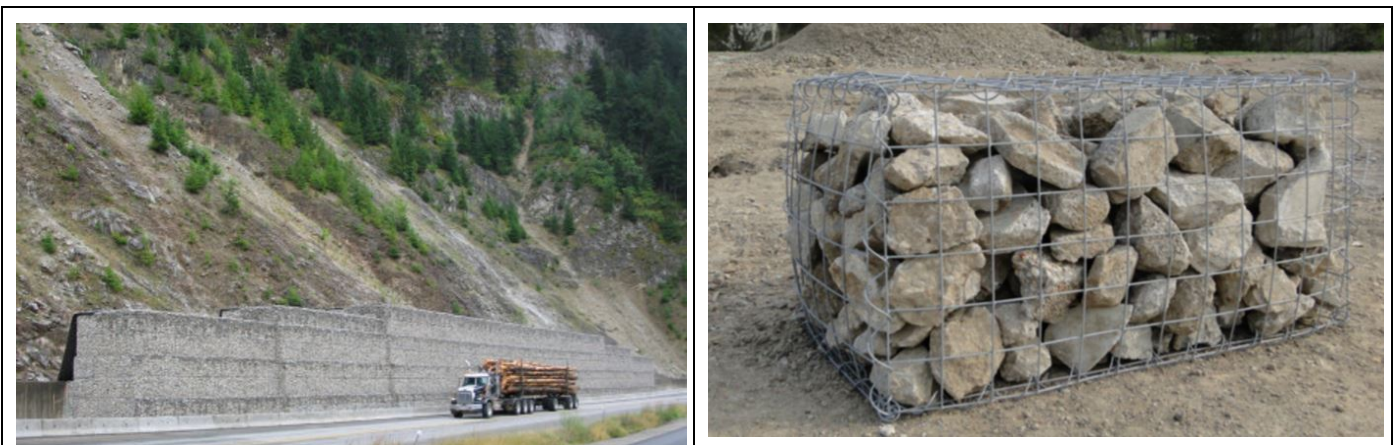
Photo 12 is an example of the extreme capability of gabion baskets utilized on a highway structure (would not be necessary for the road standard prescribed for the Prairie Creek mine). Photo 13 is typical gabion basket.
