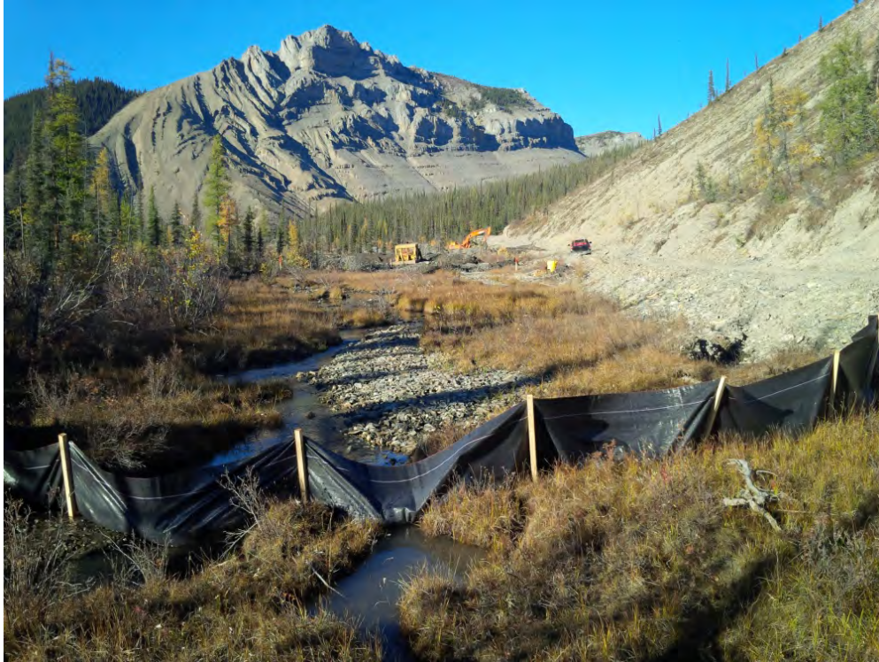
Looking north from lower silt fence. Cat is excavating South Pond and backhoe is excavating North Pond
