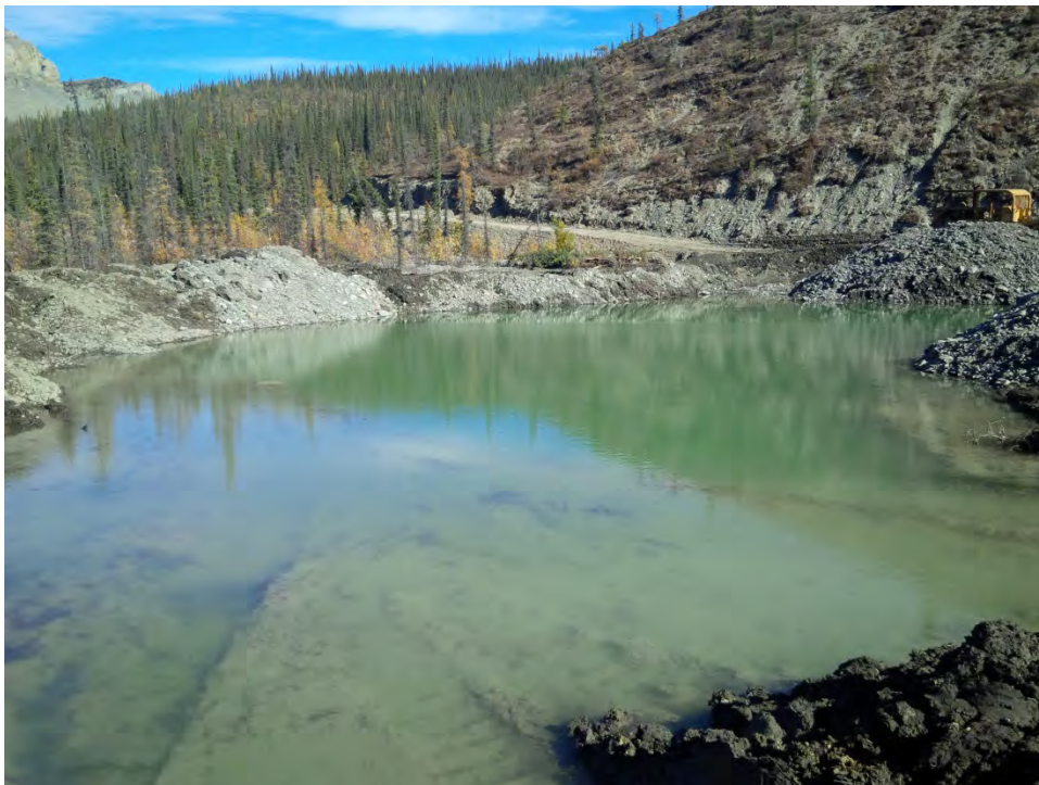
North Pond: September 13 th , showing rapid settling and clearing of pond
