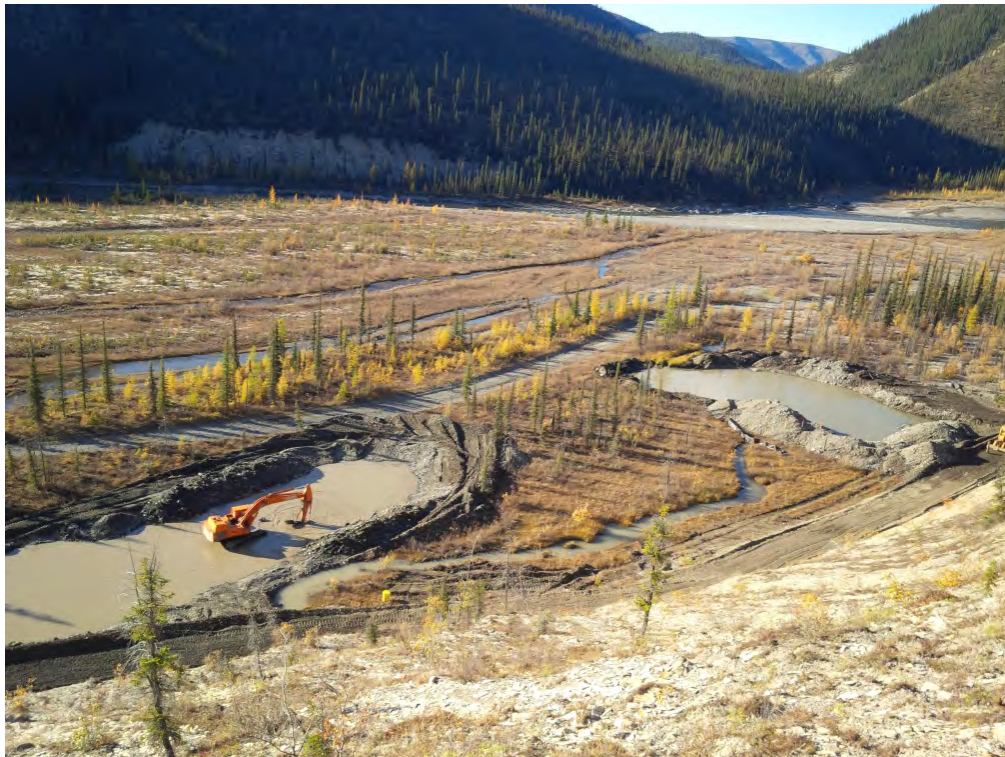
Completed North Pond and back hoe working in South Pond, both self-contained
