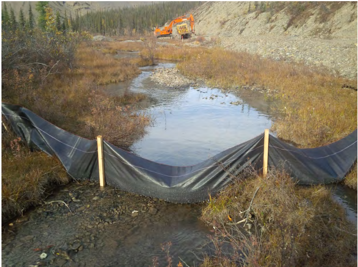
Silt fence erected downstream from South Pond Site prior to excavation
