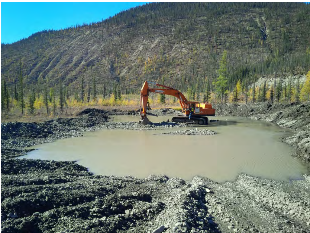
Construction of North Pond. Notice the pond is self-contained and retaining all silt
