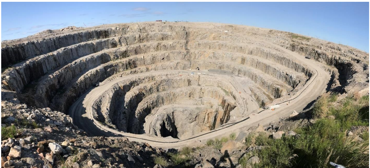
Figure 15: Pit A418, Diavik's preferred disposal location for PK, Diavik Diamond Mine Review Board photo (2019)
