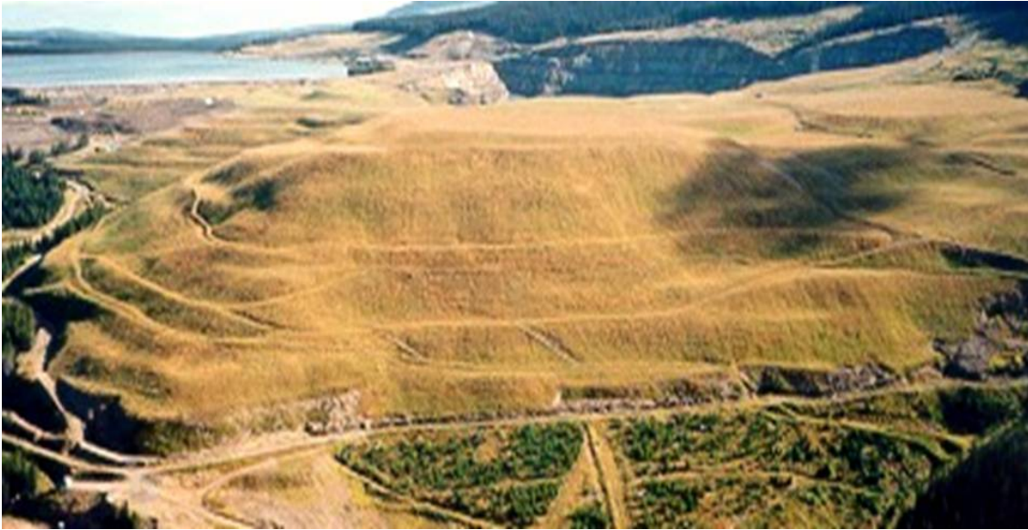
Figure 3.9 Many key properties and processes, such as weathering of mine wastes under this soil cover at the Equity Silver Mine, are difficult to measure let alone predict. (photo of Equity Silver Mine in northwest British Columbia from Mike Aziz, Goldcorp Canada Ltd.).
