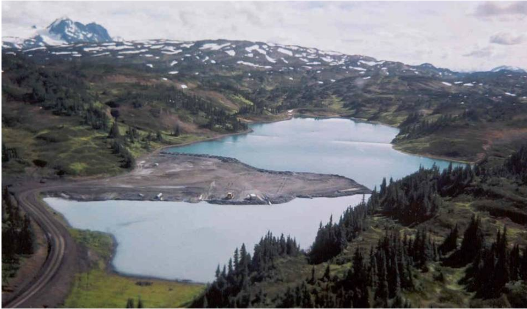
Figure 4.4c During mining, prediction also includes monitoring weathering prior to mitigation (in this case flooding) and the volume and chemistry of the associated drainage (photo of Eskay Creek Mine in northwest British Columbia).
