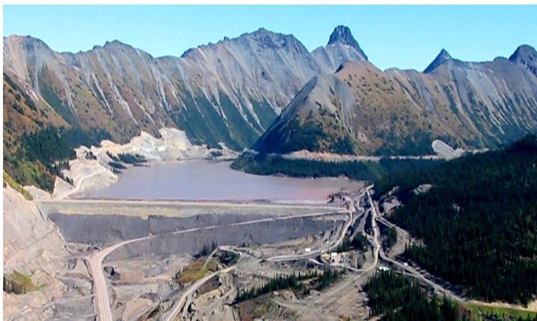
Figure 4.4b Characterization of rock quarried next to the tailings dam at Kemess South, a considerable distance from the mine, indicated it was potentially net acidic and therefore unsuitable for dam construction (photo from Harold Bent, Northgate Minerals Ltd.).
