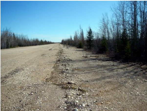
Photo 3: View of existing haul road at the historical Pine Point Mine site.
